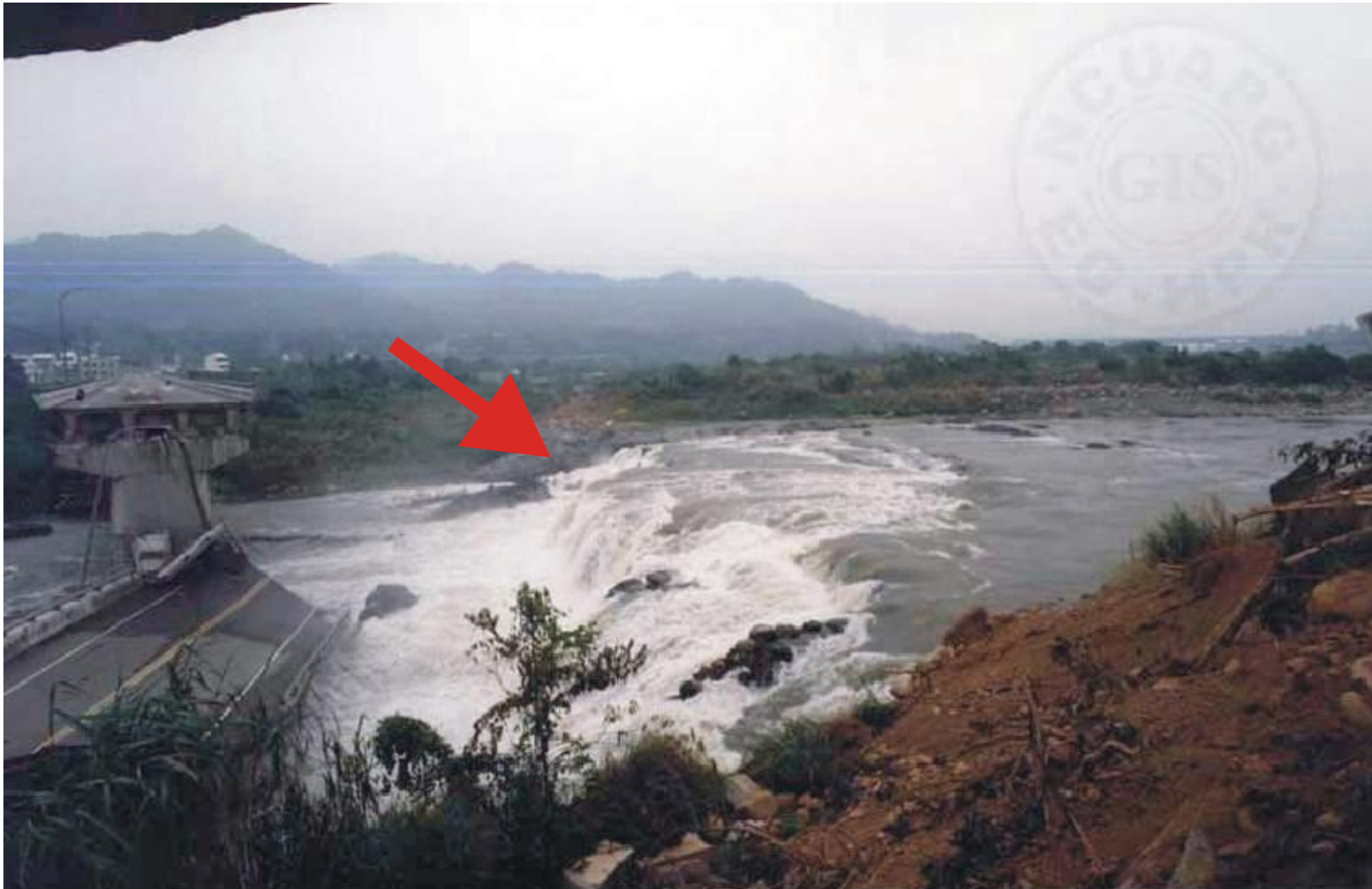
8 m vertical ground displacement, Chi-Chi Taiwan earthquake ( M_w 7.6 )
